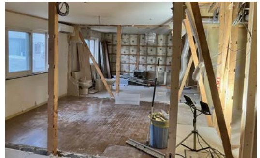
Before (Apartment walls removed)
